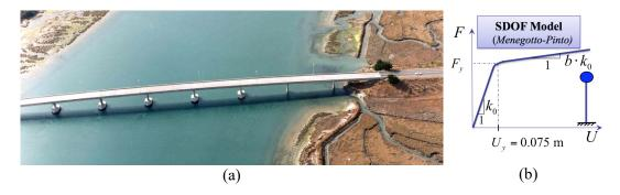
**Figure 4:** Humboldt bay middle channel (HBMC) bridge (courtesy of Caltrans): (a) isometric view, and (b) simplified nonlinear SDOF model to represent the longitudinal nonlinear response behavior of the bridge
